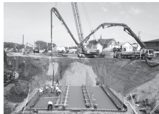
Pouring concrete for the floor of the triple box culverts at Garfield Avenue.
