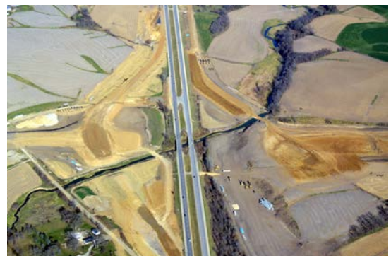
Southwest Arterial / US20 Interchange Grading Underway
