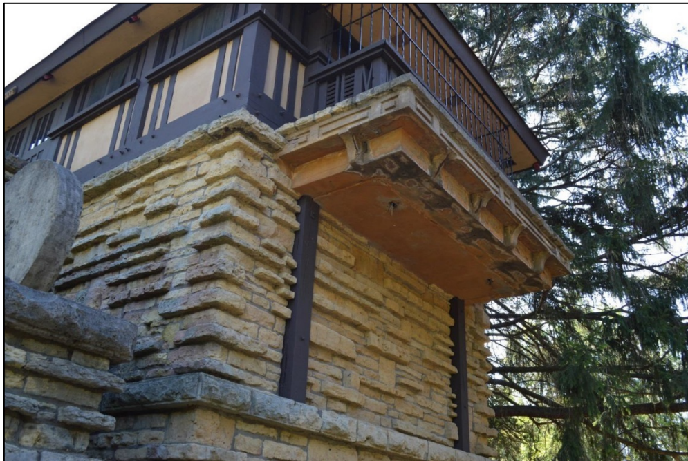
FIGURE 6 Detail of the western end of the Bridge Complex, showing the deterioration of the balcony and its missing lighting fixtures. Source: Photograph by Dr. Julie Schlarman September 14, 2015.
