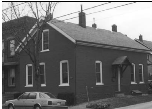
Figure 169: 2307 White Street (pre-1884) (photo by Jim Jacobsen, March 7, 2000)
