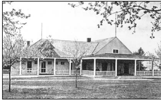
Figure 183: Pre-bungalow, described as a “low rambling building, all with wide porches and low windows,” the Dubuque Golf Club clubhouse ( Enterprise , June 18, 1904)
