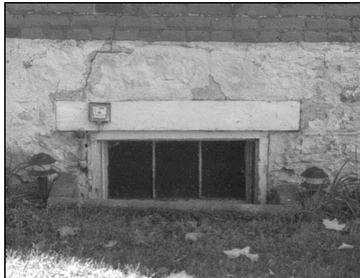
Figure 153: Wooden lintel, stone foundation window
