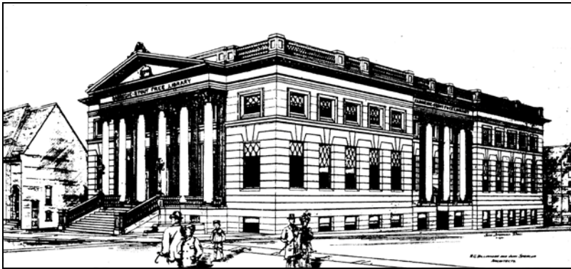
Figure 196: Carnegie-Stout Public Library, 11 th & Bluff streets, W. G. Williamson, Architect Temple Front type, Neoclassical style, 1901
