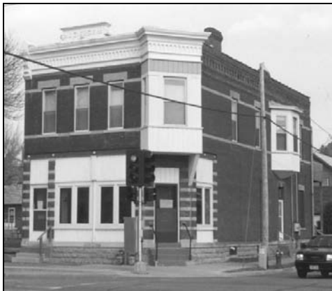
Figure 250: 2600 Jackson Street (1903) (photo by Jim Jacobsen, March 7, 2000)
