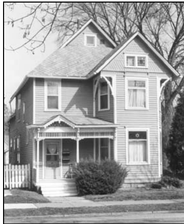
Figure 108: 2568 Jackson Street (1900) (photo by Jim Jacobsen, March 7, 2000)
