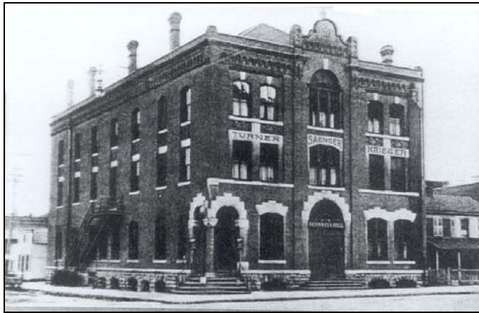
Figure 227: Turner/Germania Hall, 9 th & Iowa, southeast corner 1892 (non-extant) (Center For Dubuque History, Loras College, Photo GRS #3469) (Two-part commercial block type)
