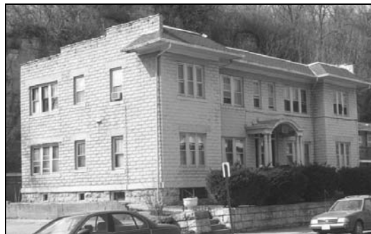
Figure 148: 2555-65 Central Avenue (1923) (photo by Jim Jacobsen, March 7, 2000)
