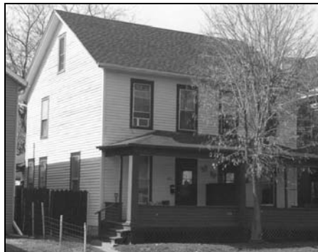
Figure 173: 2255-57 Central Avenue (1884) (photo by Jim Jacobsen, March 7, 2000)
