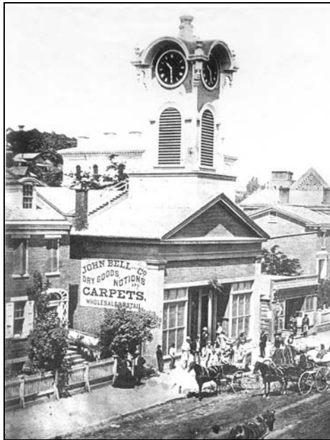
Figure 203: First Clock Tower Building, a former Congregational church (built 1845, collapsed 1872), west side Main north of 8 th , c.1872. This was a temple front converted for store use and any Italianate style linkage is derived from the addition of the clock tower.
