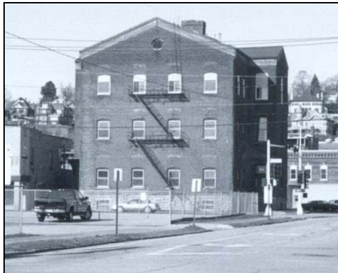
Figure 75: Third Ward/Prescott School (12 th and Central streets, 1857, John Rague, architect) (photo by James Jacobsen, April 21, 2000)
