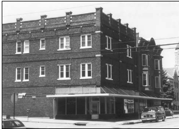
Figure 243: 1103-13 Central Avenue, view northwest, c.1915 (photo by J. Jacobsen, May 2003)
