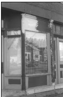
Figure 155: 2311 Windsor, stone lintel line, storefront
