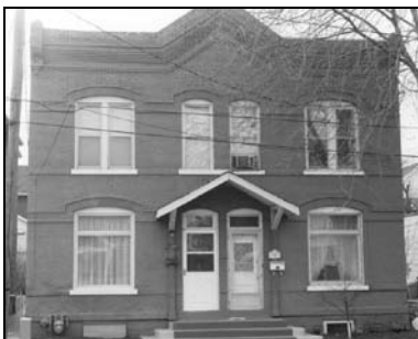
Figure 189: 2255-57 Jackson Street (1891-92) (photo by Jim Jacobsen, March 7, 2000)
