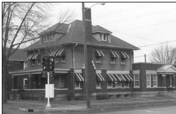
Figure 147: 2006 Jackson Street (1909) (photo by Jim Jacobsen, March 7, 2000)
