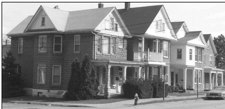
Figure 129: 2590, 2586-88, 2582, 2578 Central Avenue (1915-25) (photo by Jim Jacobsen, March 7, 2000)
