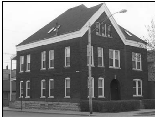
Figure 121: 2070-72 Jackson Street (1891-1909) (photo by Jim Jacobsen, March 7, 2000)
