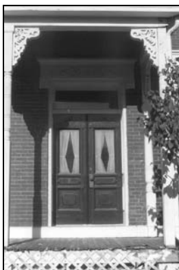
Figure 156: Original double doors, transom and carved stone lintel and porch detailing
