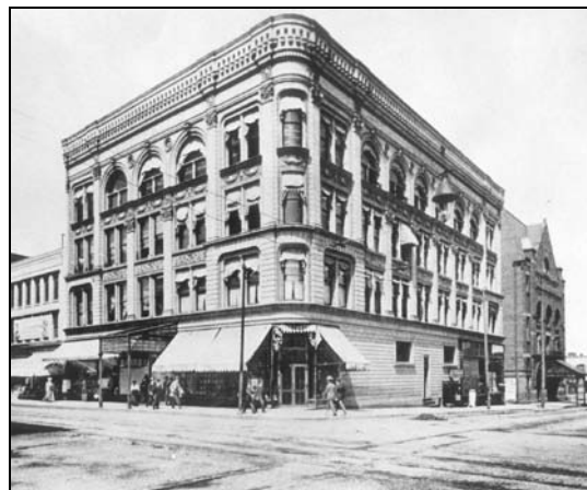
Figure 233: Security Building, 1896 (courtesy Loras College) (Stacked Vertical Block type)
