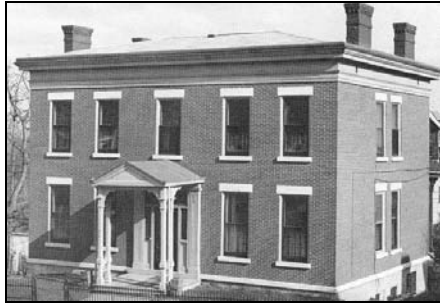
Figure 58: 710 Fenelon Place (photo, Sommer, p. 135)
