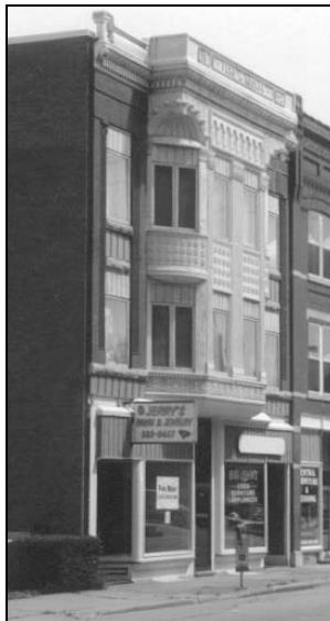
Figure 221: Fred A. Nesler Block, 1732-36 Central Avenue, 1892, view southeast (photo by J. Jacobsen, November 2002)
