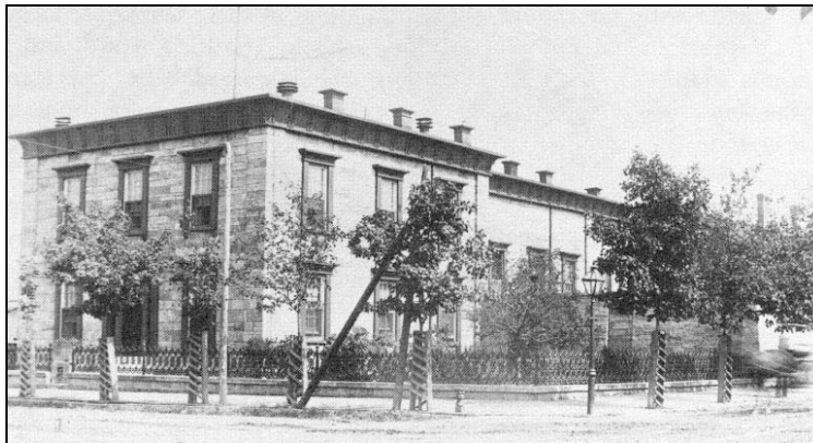
Figure 84: Former Dubuque County Jail, 36 East 8th Street (1857-58) façade to left, view southeast (photo, Horton, "Early Architecture in Dubuque," p. 141)
