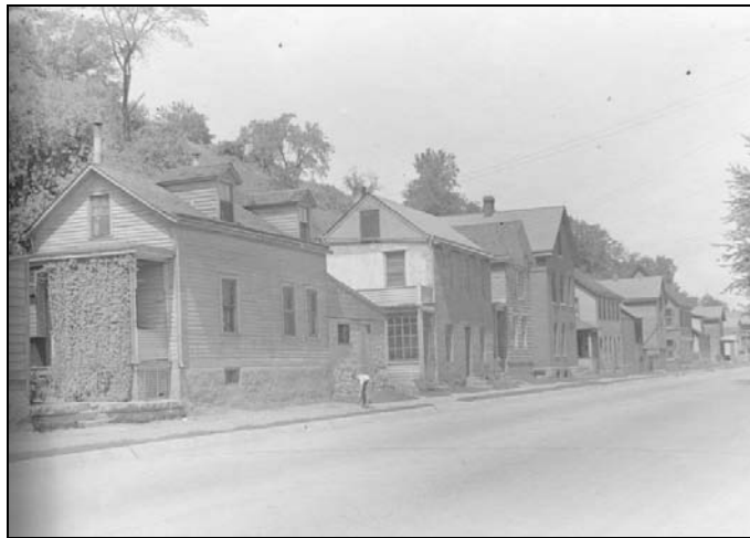
Figure 45: Intermixed brick and frame houses, stone foundations, likely Central Avenue ( Housing and Health Survey, 1934 )
