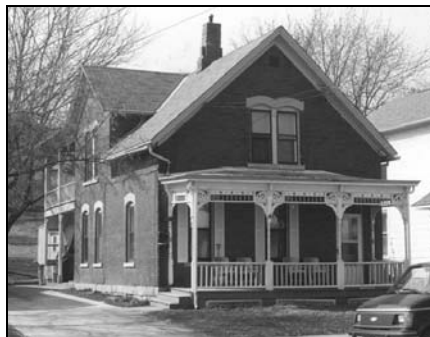
Figure 162: 2461 Central Avenue (1890) (photo by Jim Jacobsen, March 7, 2000)
