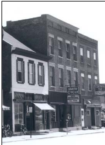
Figure 212: 1056 Central Avenue (center, view southeast) (Photo by J. Jacobsen, May 2003)
