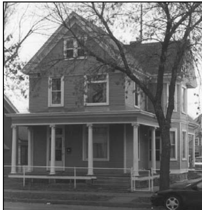
Figure 131: 2044 Jackson Street (1900) (photo by Jim Jacobsen, March 7, 2000)
