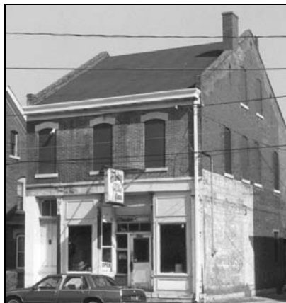
Figure 60: 2306 Central Avenue (1881) (photo by Jim Jacobsen, March 7, 2000)
