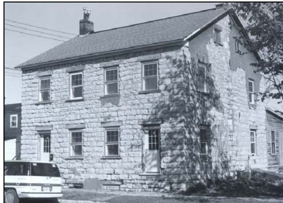
Figure 48: Stone double house, East 14 th and Maple, view northwest (photo by James Jacobsen, April 21, 2000) The rear wing might be of log construction.
