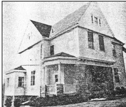
Figure 127: 514 Fenelon Street (c.1910) (photo, A Walking Tour...South Dubuque)
