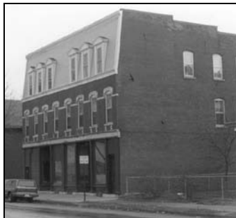
Figure 94: 1913-17 Jackson Street (1886) (photo by Jim Jacobsen, March 7, 2000)
