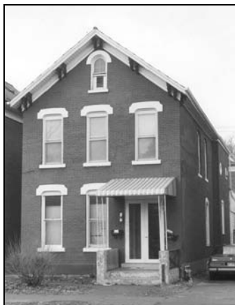
Figure 80: 1815 Jackson Street (1884-91) (photo by Jim Jacobsen, March 7, 2000)
