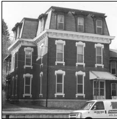
Figure 93: 2133 Central Avenue (1884-1890) (photo by Jim Jacobsen, March 7, 2000)
