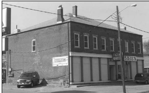
Figure 63: 2327 Central Avenue (1855) (photo by Jim Jacobsen, March 7, 2000)
