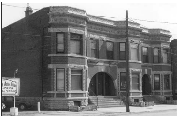
Figure 142: 2130-34 Central Avenue (1891-1902) (photo by Jim Jacobsen, March 7, 2000)
