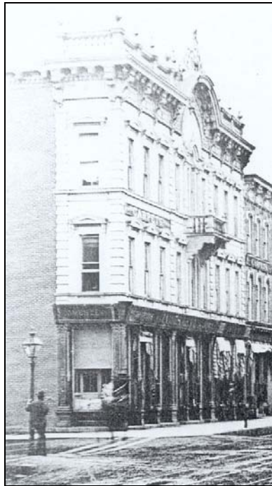
Figure 213: 576-98 Main Street, c.early 1880s (Center For Dubuque History, Loras College, Photo Ham House-#843) (Two-part commercial block type)
