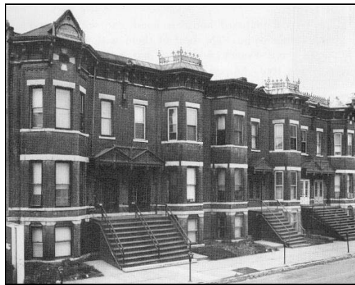
Figure 83: 975 Locust Street (photo, Sommer, p. 91)
