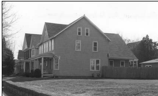
Figure 175: 2523 Central Avenue (1892-1909) (photo by Jim Jacobsen, March 7, 2000)
