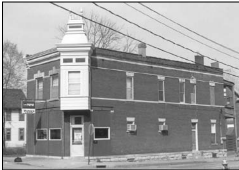
Figure 249: 2600 Central Avenue (1898) (photo by Jim Jacobsen, March 7, 2000)
