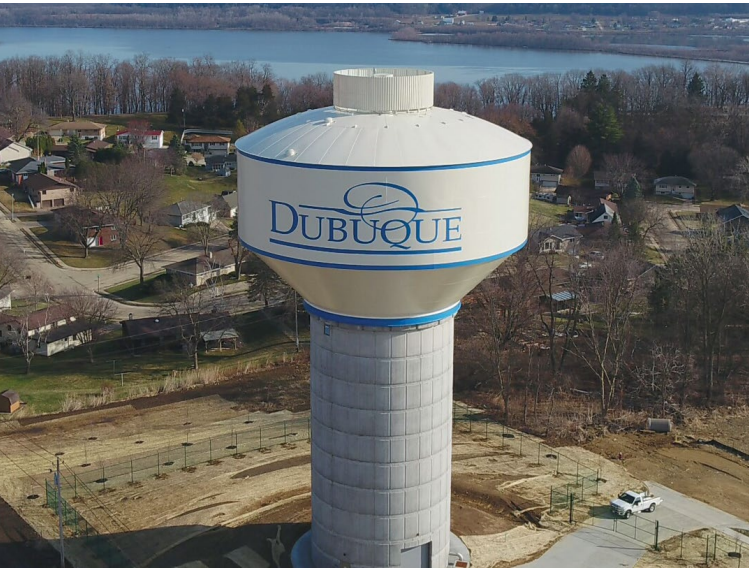
Roosevelt Street Water Tower Completed in 2020, the 1.25-million gallon elevated tower, along with distribution improvements, increased water pressure to customers in and around the Roosevelt Street and Peru Road area.
