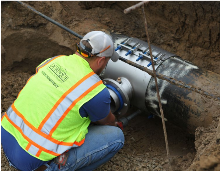
City water distribution workers tapping a water main on Cedar Cross Rd.
