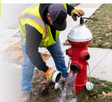
The Water Department will conduct fire hydrant flushing throughout the spring and summer months. Flushing is essential for preserving the water system's integrity and maintaining an adequate water supply for Dubuque households and firefighting.
