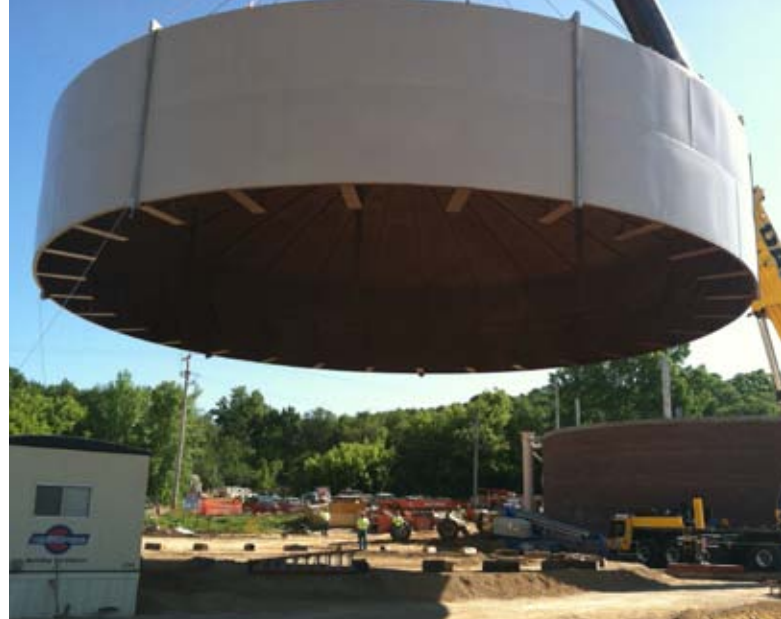
// A crane prepares to lower a lid onto one of the anaerobic digesters //
