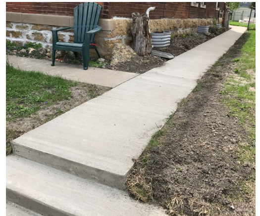
The existing sidewalk was removed and replaced at an adequate slope to facilitate drainage away from the house.
