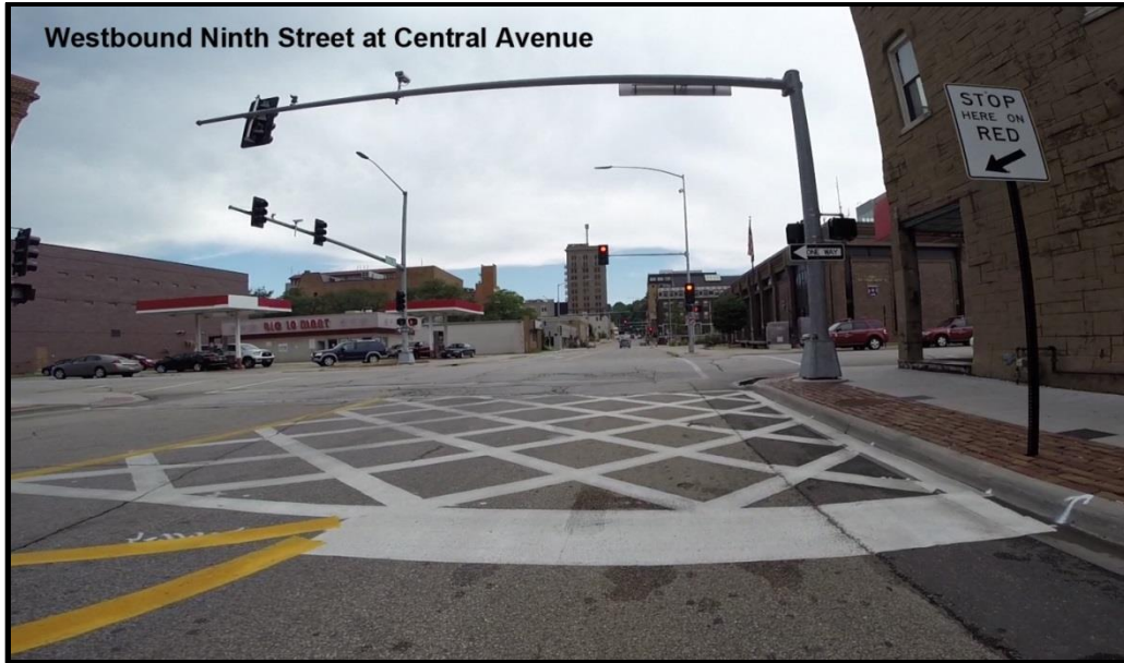
Two Intersections on Ninth Street Feature the Crosshatch Markings
