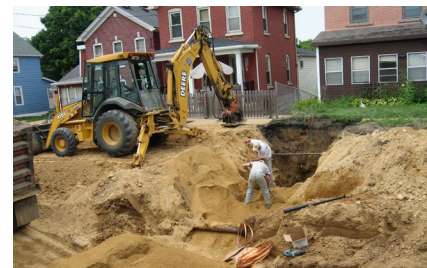
WATER MAIN REPLACEMENT
