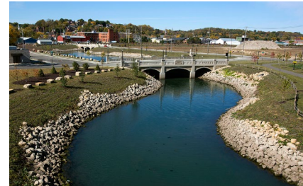
BEE BRANCH FLOOD MITIGATION
