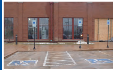
The correct way (above). This is an example of maximum accessibility with curb-cut access, posted signs at sufficient height, and stenciled icons (not required) for each space.
