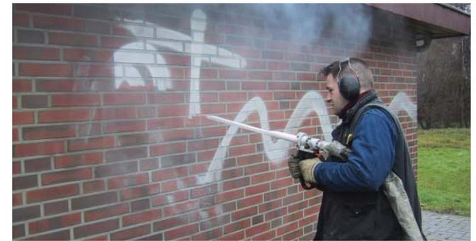
Generally, abrasive cleaning methods are not acceptable for use on historic masonry buildings because they remove a portion of the surface, instead of cleaning it.
