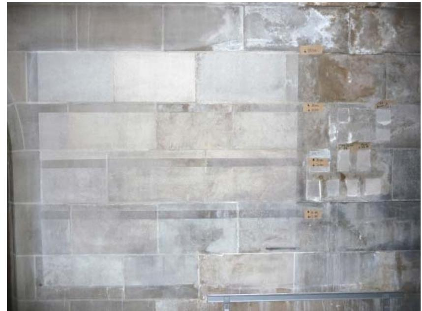
CAUTION -The examples listed below are considered appropriate cleaning methods for the masonry type listed, but may NOT be the best way to clean every building. Each building and material is unique, so testing must be done to determine the most effective, gentlest cleaning method that should be used.
