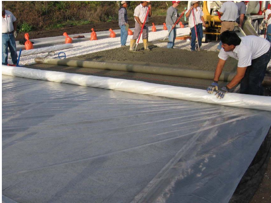
Figure 11: Covering fresh pervious concrete with plastic for 7 day moist curing period (ISU Lot 122, 2006)
