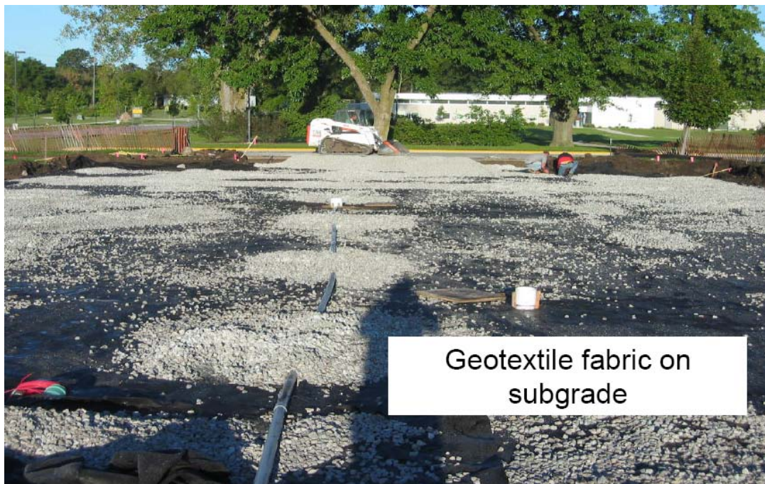
Figure 2: Placement of geotextile and aggregate subbase on subgrade (Lot 121, Iowa State University, 2007)
