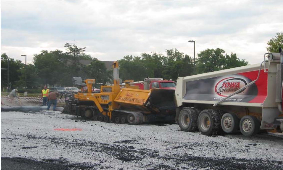
Figure 4: Placement of porous asphalt material (Lot 121, Iowa State University, 2007)
