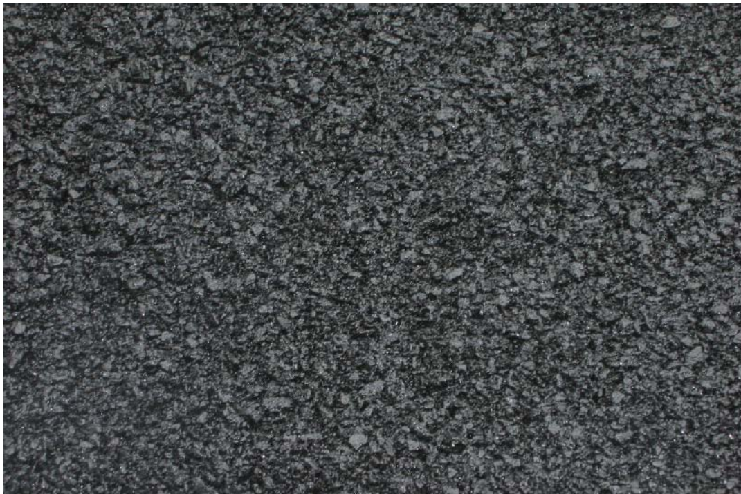
Figure 6: Finished porous asphalt surface (18% porosity, PG 82-22) (Lot 121, Iowa State University, 2007)
