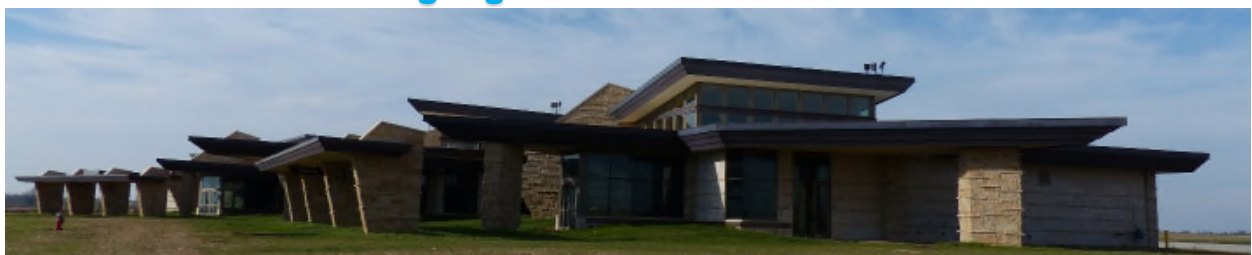
New Terminal Facility Currently Under Construction – Scheduled Opening 2016
