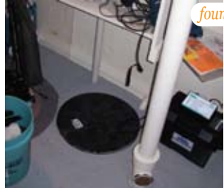
foundation drain to sump pit - PROPER
