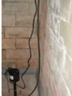
flex hose to outside - IMPROPER
