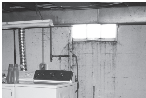
Leaking basement windows.
