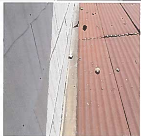
D-17: Tar on lean to flashing to building 3, on metal and transite
