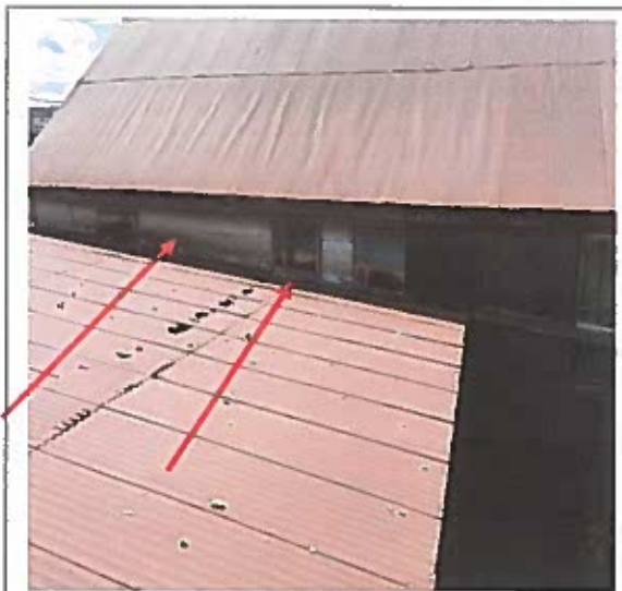
D-17: Tar on lean to flashing to building one and three.
