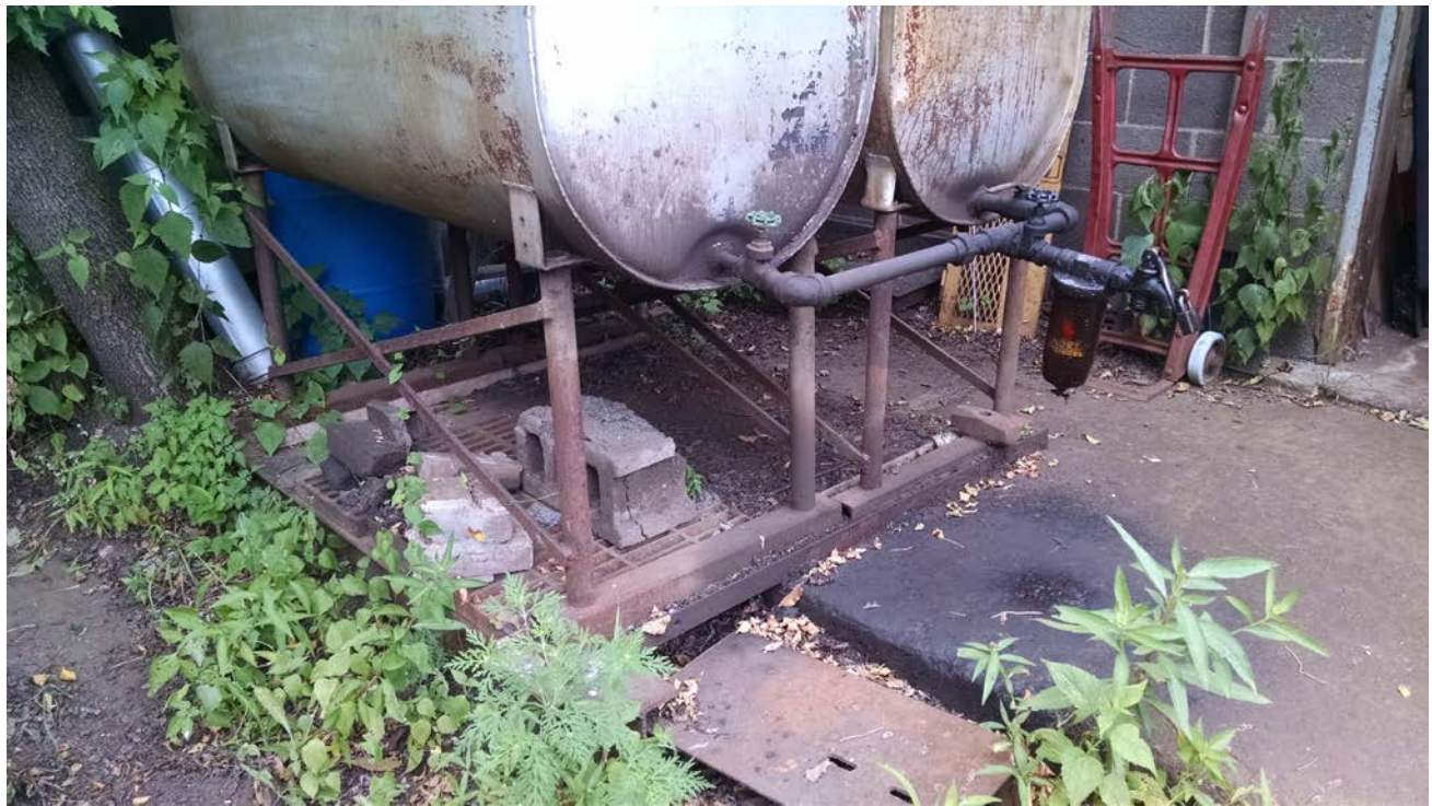
Photo 19 – View of two ASTs and staining located outside the control building on the grounds of the west side property.
