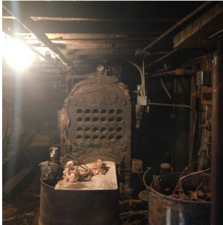
Photo 3 – Steam boiler wrapped in fiberglass insulation in basement in the main office building.
