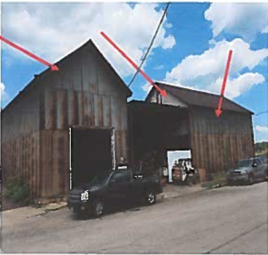
D-3: Transite siding under metal, top half of buildings.
