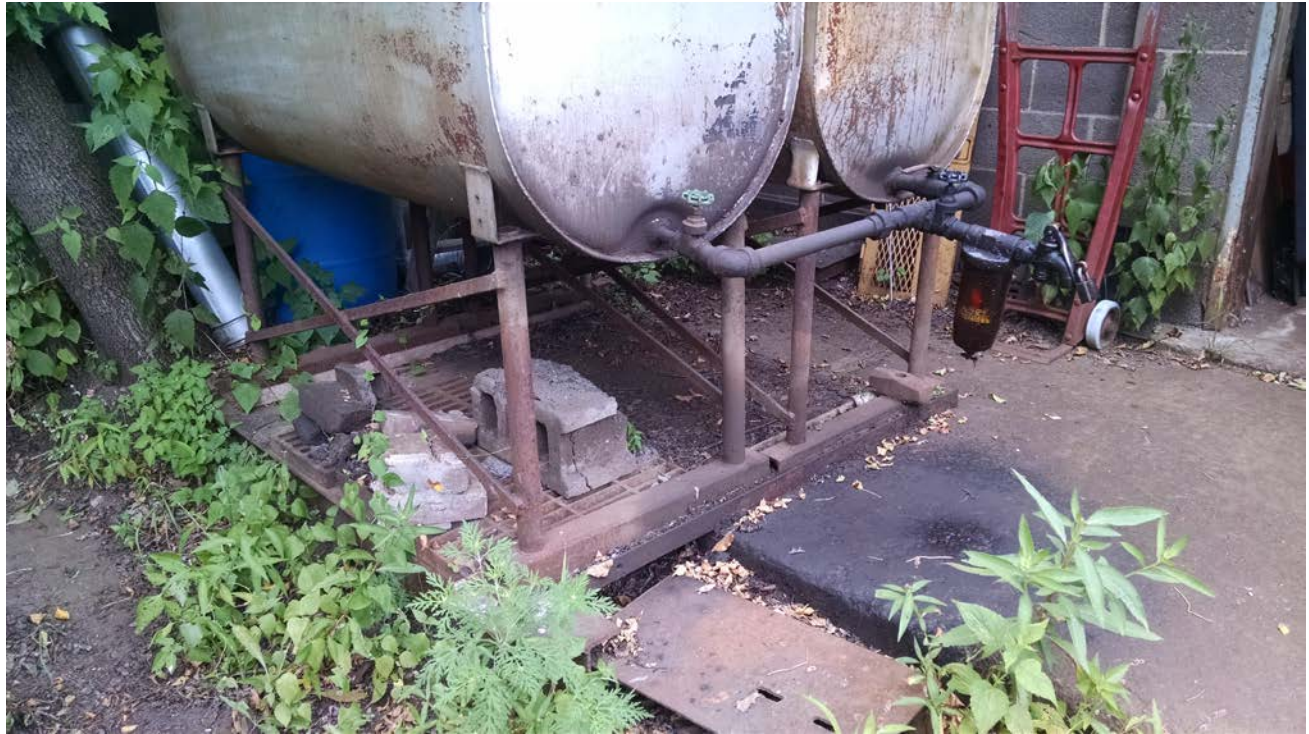
Photo 19 – View of two ASTs and staining located outside the control building on the grounds of the west side property.
