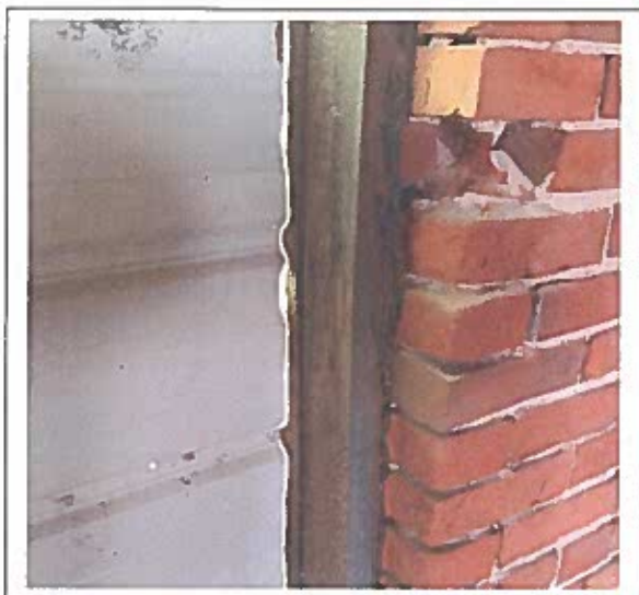
A-35: Caulking interior windows (mainly 4 th floor) wood frame to brick Elm St. building.
