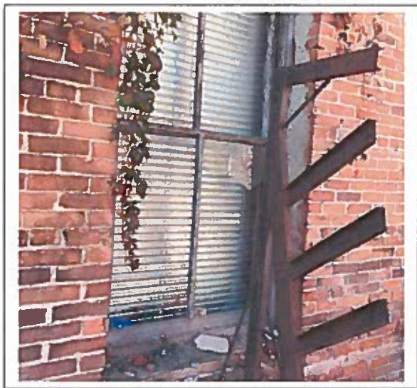
A-15: Window glazing, old wood frames along Elm Street wall, covered by metal on the outside of the building.
