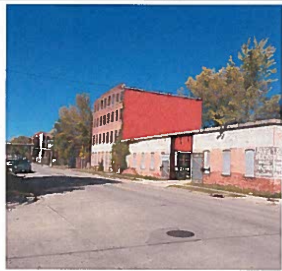
Elm St Four Story Building, and front wall
