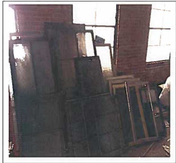
Stock piled windows with glazing, assumed positive.
