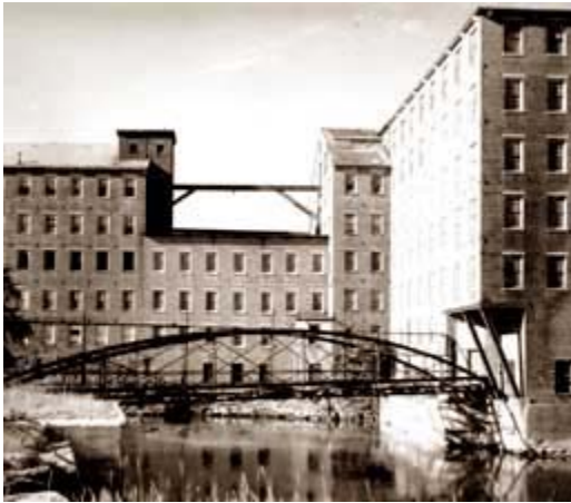
Windows are frequently important visual focal points, especially on simple facades such as this mill building. Replacement of the multi-pane windows with larger panes could dramatically alter the appearance of the building. Photo: NPS files.
