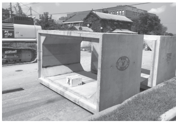
New precast concrete storm sewers before installation in August 2018.
