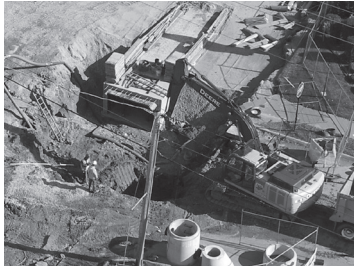
A new concrete storm sewer is installed along 22nd St. in October 2018.
