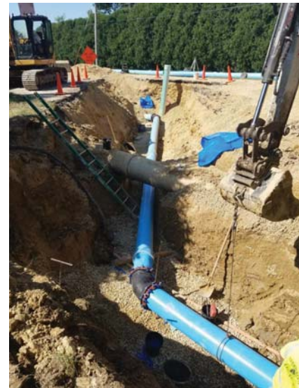
JFK Road Water Main Installation FY18
