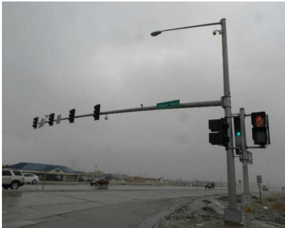
Intersection with microwave traffic detectors uninhibited by extreme weather conditions
