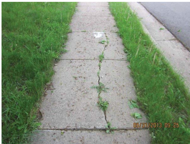
Cracked and heaving sidewalk - Tripping hazard
