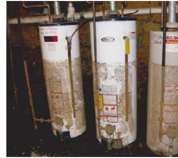
Basement flooding high water mark on water heaters
