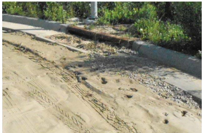
Sediment deposition clogging a storm sewer inlet
