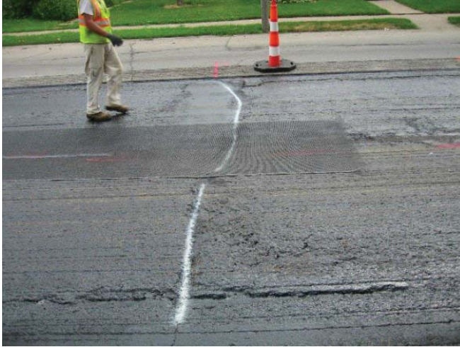
Installation of Geogrid over joints
