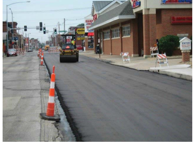
New Asphalt Interlayer Installation to reduce cracking
