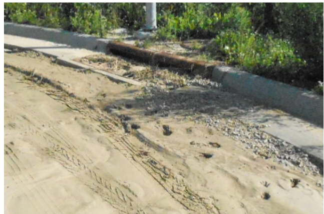
Sediment deposition clogging a storm sewer inlet
