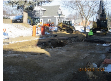
Emergency Water main repair in the winter
