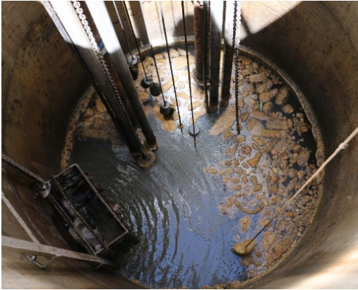
Oils and grease in a sanitary sewer lift station
