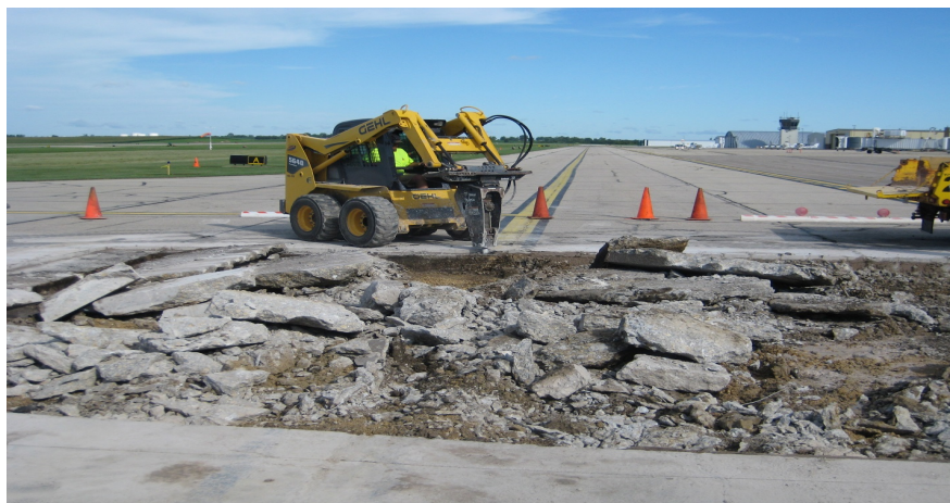
Airport staff work on replacing an area of concrete on a taxiway
