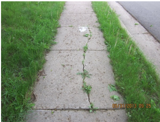
Cracked and heaving sidewalk - Tripping hazard
