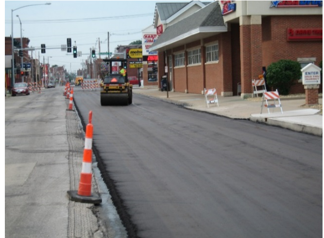
New Asphalt Interlayer Installation to reduce cracking
