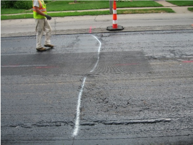
Installation of Geogrid over joints
