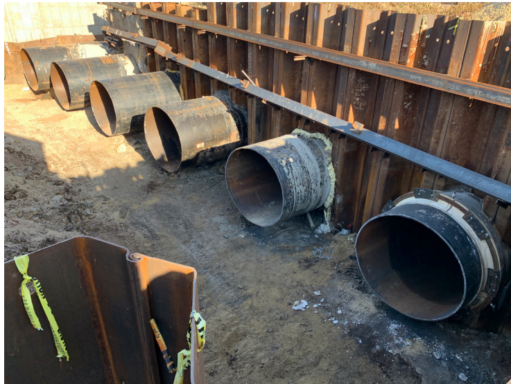
The installation of the sixth and final pipe was completed on Oct. 30. The pipes are 8-foot in diameter and approximately 200-feet long.
