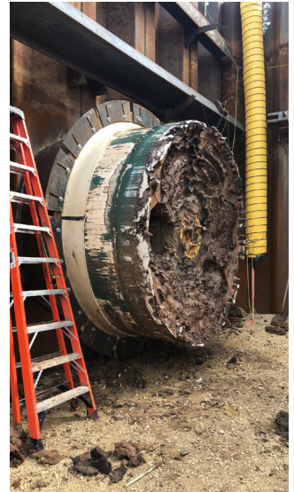
The microtunneling machine reaching the other side.
