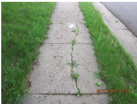
Cracked and heaving sidewalk - Tripping hazard
