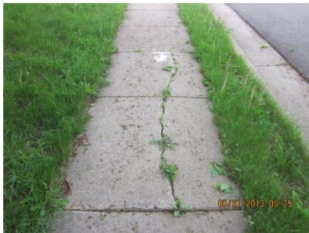
Cracked and heaving sidewalk - Tripping hazard
