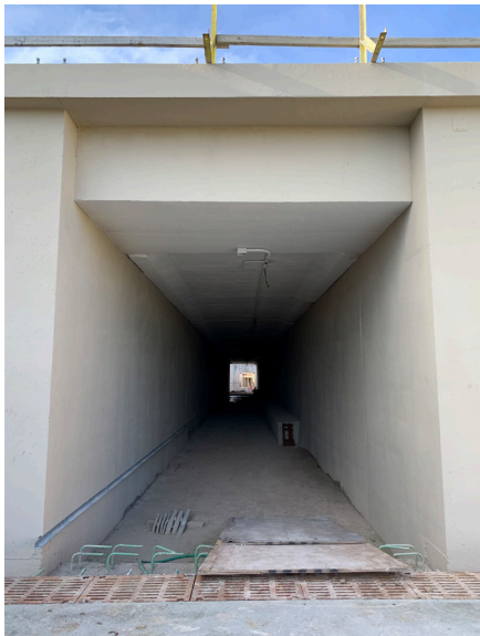
The tunnel ceilings and walls have been smoothed and painted.
