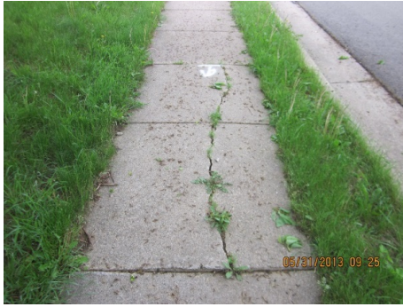
Cracked and heaving sidewalk - Tripping hazard
