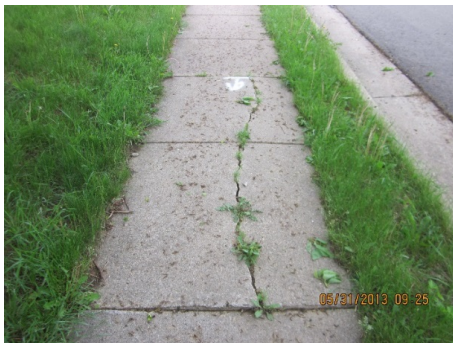
Cracked and heaving sidewalk - Tripping hazard
