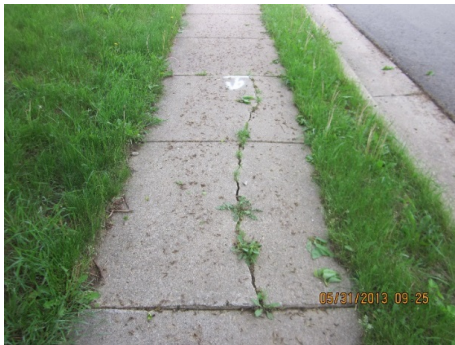
Cracked and heaving sidewalk - Tripping hazard
