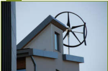
Building mounted wind turbine
